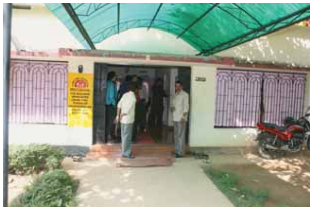
Renovation of facility in Kerala
